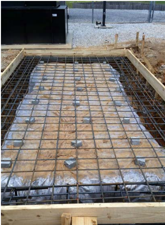
Fuel Tank Slab
